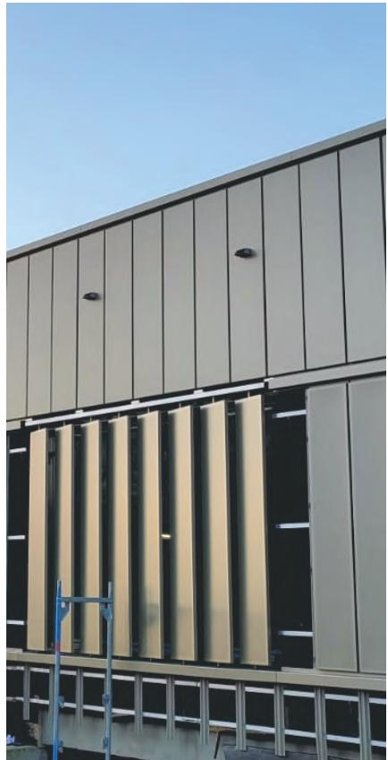
Ventilated facades combine tradition and modern technology to provide essential thermal and weather protection for buildings. They offer diverse forms and materials and are highly functional, with excellent sound insulation, fire resistance, and lightning strike resistance.
