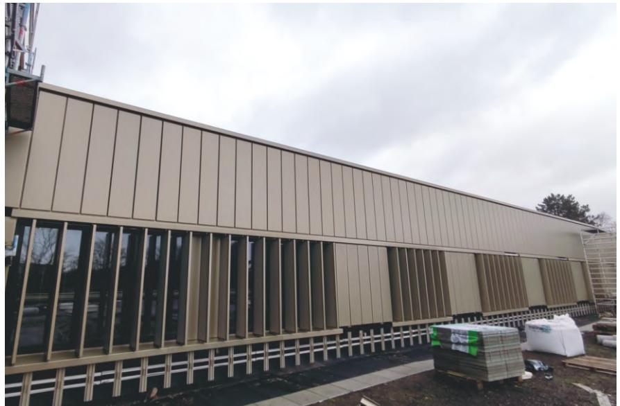
Facades are exposed to external conditions, making them crucial for preserving the internal climate. Proper planning and insulation help increase the building's energy efficiency. The construction's flexibility allows for adjusting the insulation thickness to the specific requirements of the building, making ventilated facades ideal for new projects and renovations.
